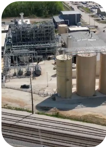
Ironton Production Plant
